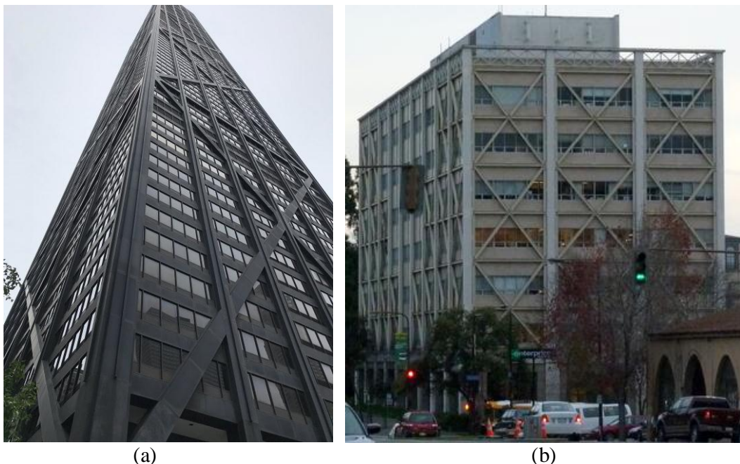
Figure 1. Examples of braced buildings: (a) John Hancock Center, Chicago, US, and (b) University Hall, University of Berkeley, California.
